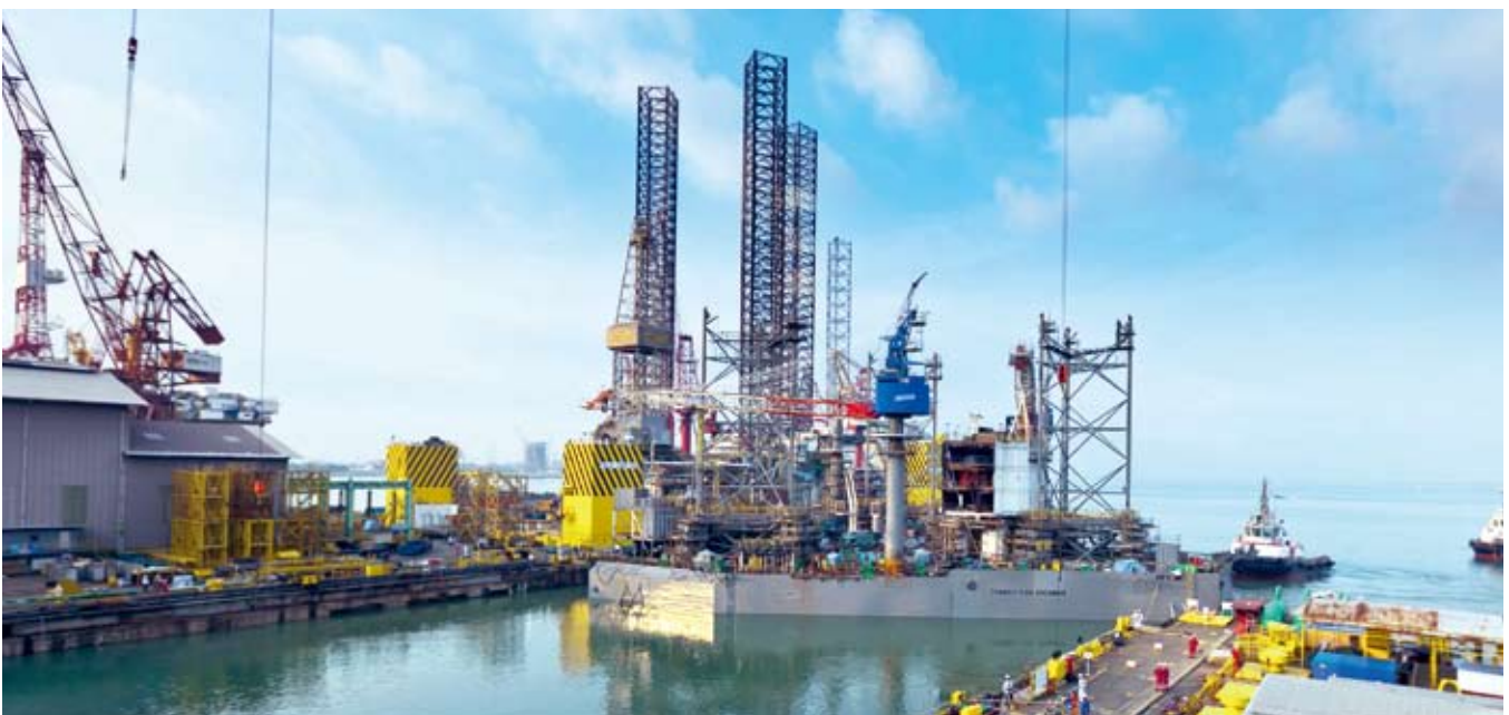
Keppel FELS' clockwork construction capability was demonstrated in its undocking of Transocean's KFELS Super B Class Big Foot jackup rigs, B326 and B327, safely and on schedule on 20 March 2012
